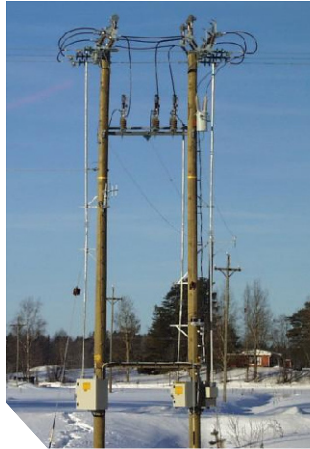
Pole-mounted disconnector from Netcontrol
